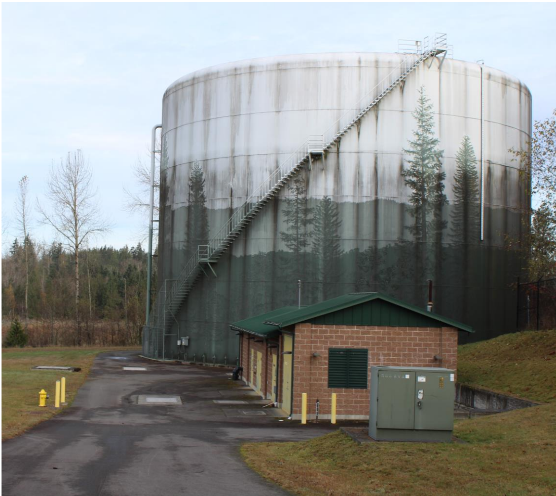
4.3 Mil Gal Water Tank
