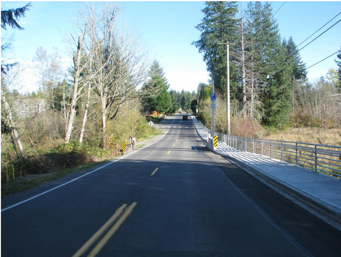
'Roberts Dr. Sidewalk and Bridge Completion'
