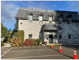
Stairs to EOC on Left
