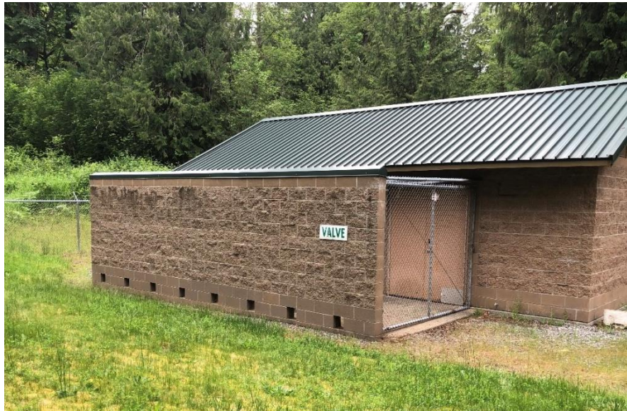
North Bank BPS (Outside)
