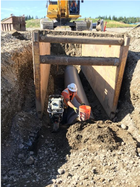
Large Diameter Water Main Installation
