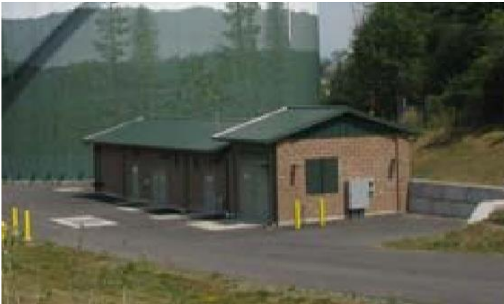
4.3 MG Reservoir Pump Station and Treatment Building
