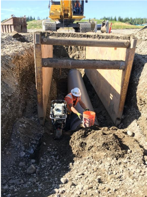
Large Diameter Water Main Installation
