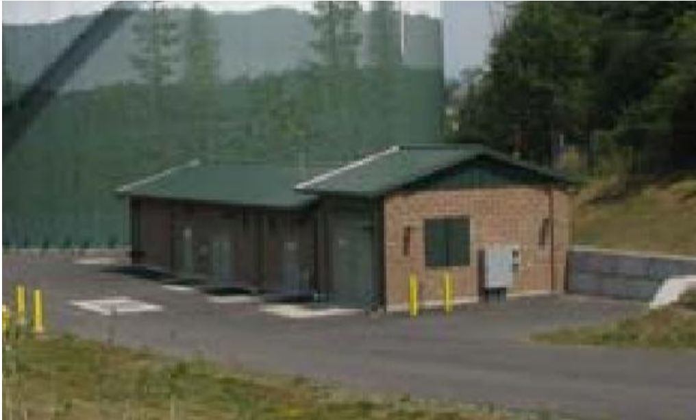
4.3 MG Reservoir Pump Station and Treatment Building
