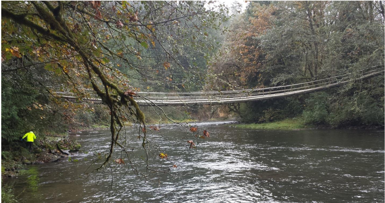
Green River Pipe Bridge
