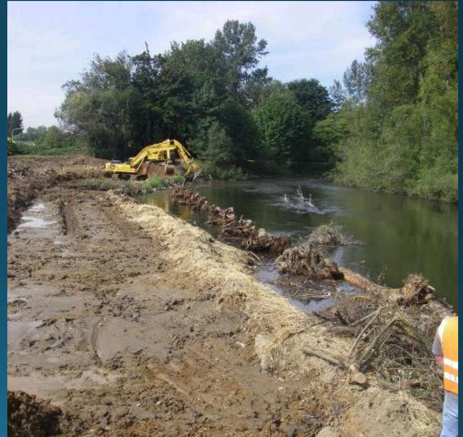
Fenster Levee Setback, Auburn
