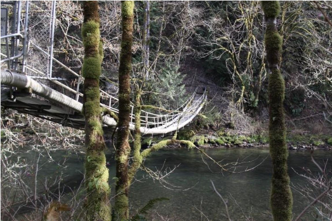
‘Swinging Bridge Leading to the Springs Water Source’
