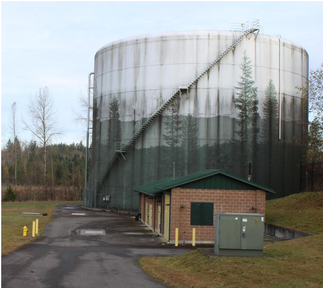
4.3 Million Gallon Water Tank
