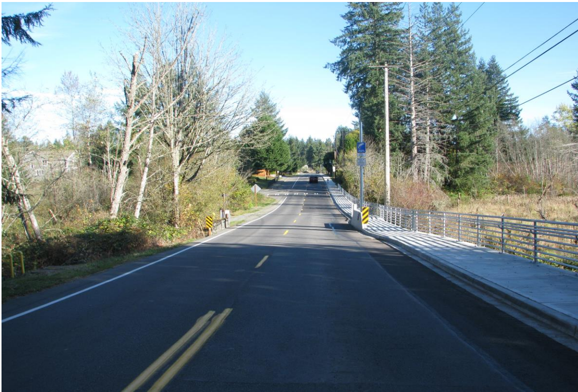
‘Roberts Dr. Sidewalk and Bridge Completion’
