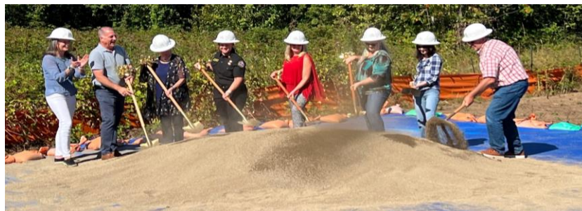
Breaking Ground for the New Fire Station
