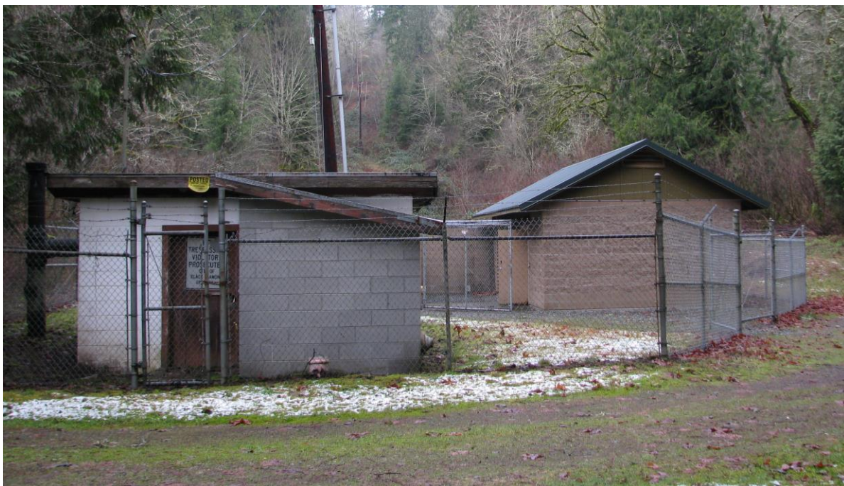
'Pump Station Building'
