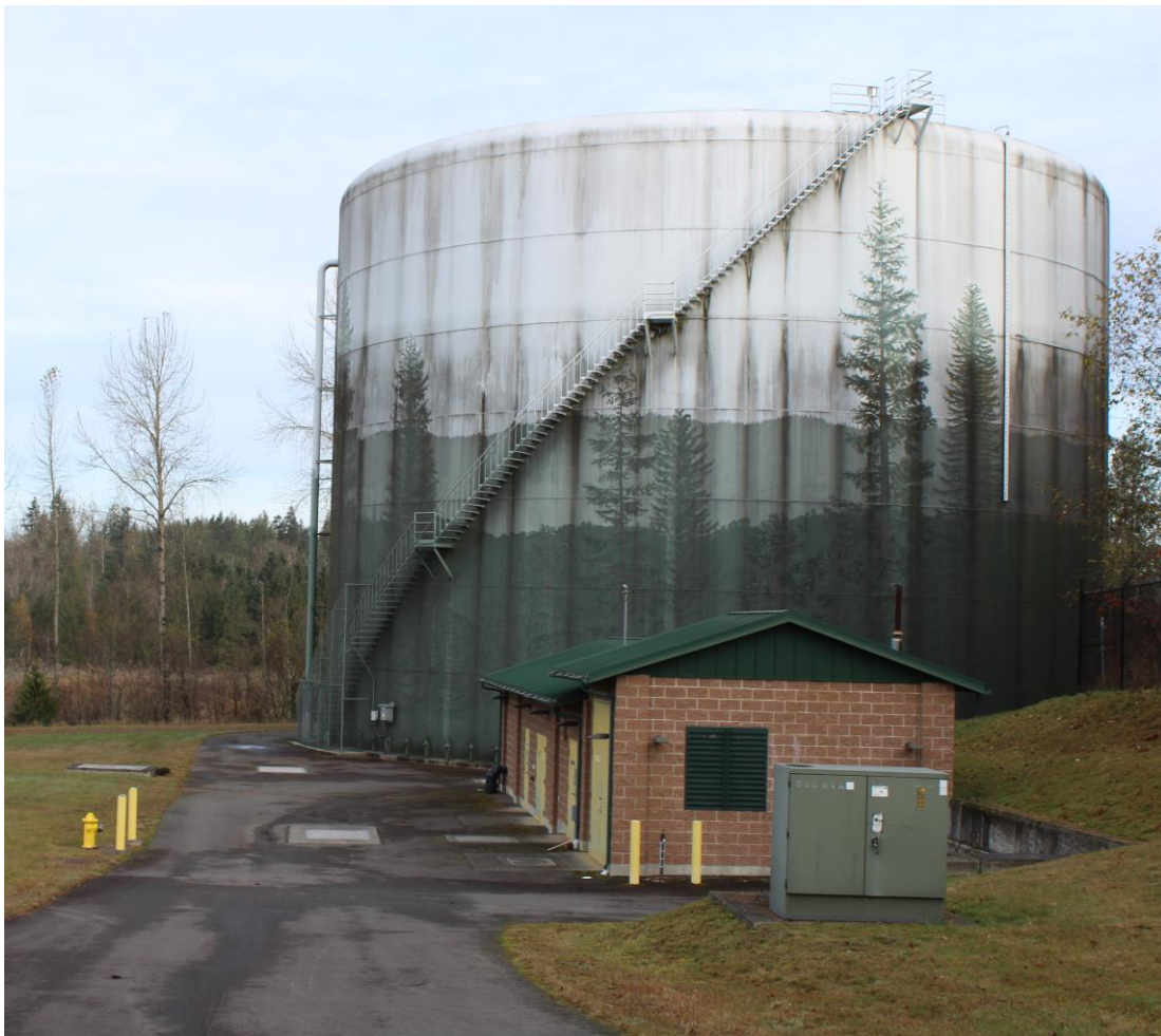
‘4.3 Mil Gal Water Tank’
