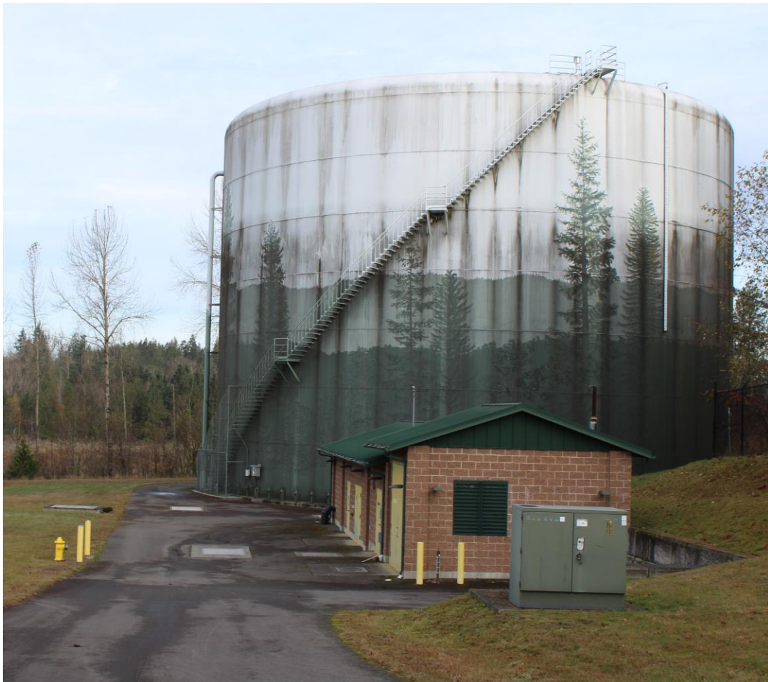
4.3 Mil Gal Water Tank
