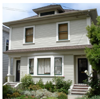
Duplex Stacked 2 units
